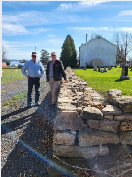
The completed east wall with widened roadway & the north wall requiring work along with Walter MacLean and Mick Bettany.
