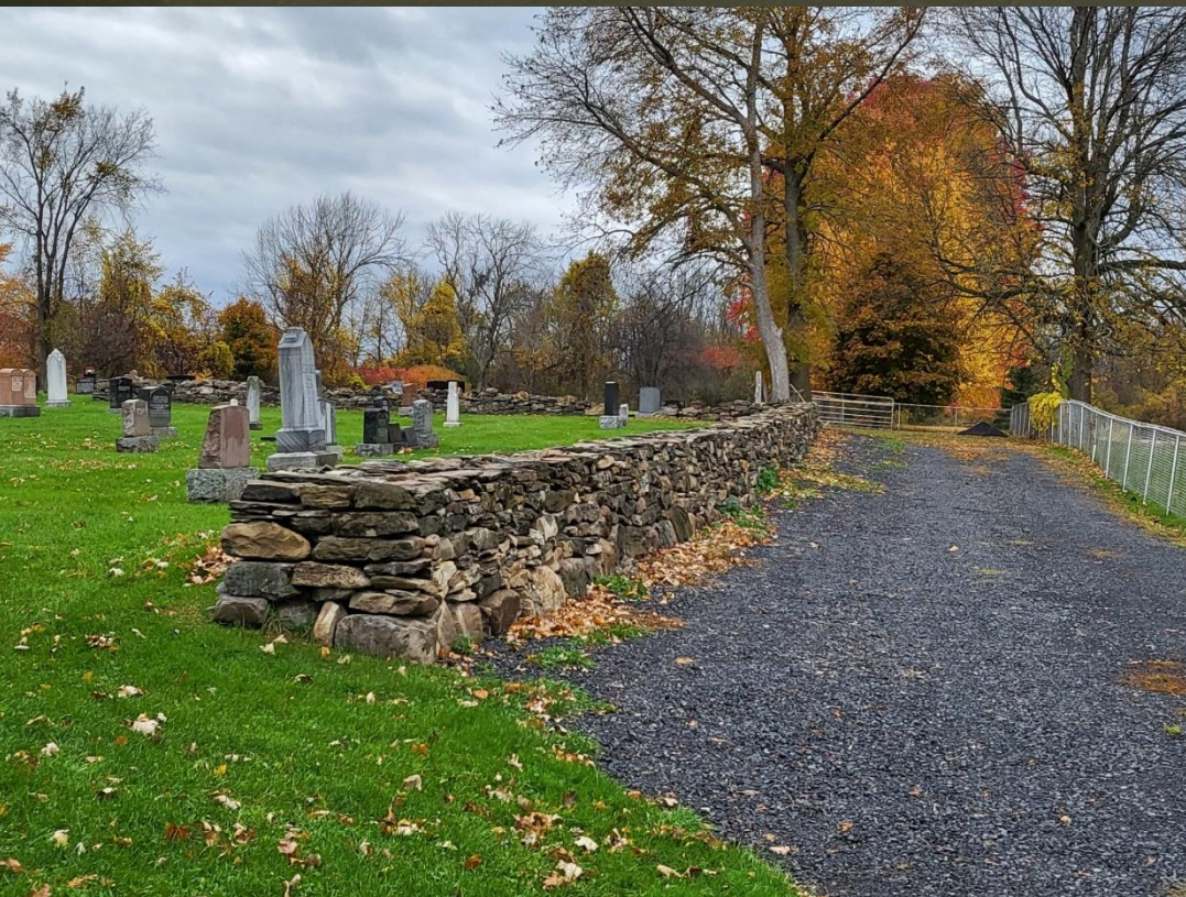
Completed work – east wall
