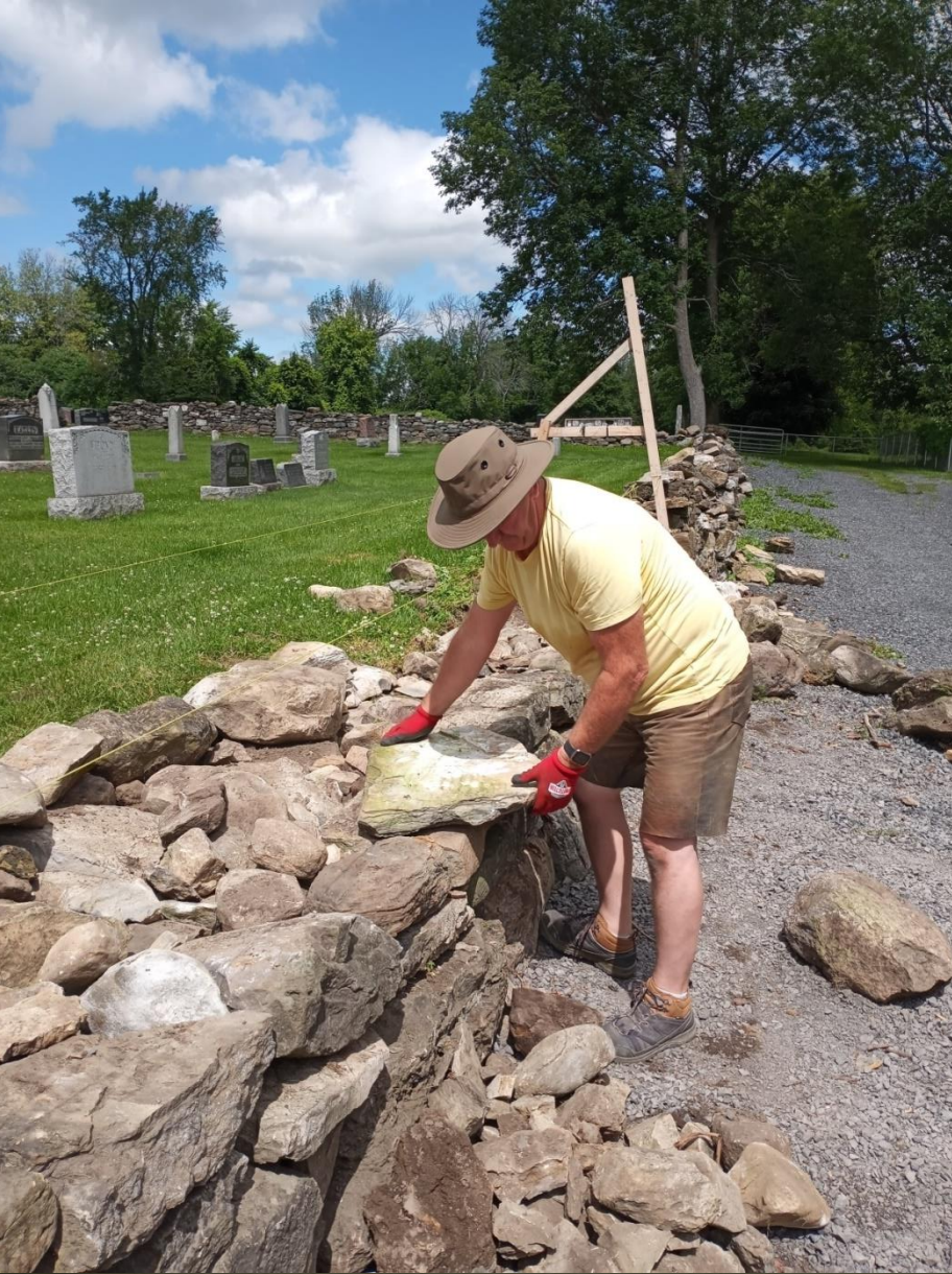
Mick working on the east wall
