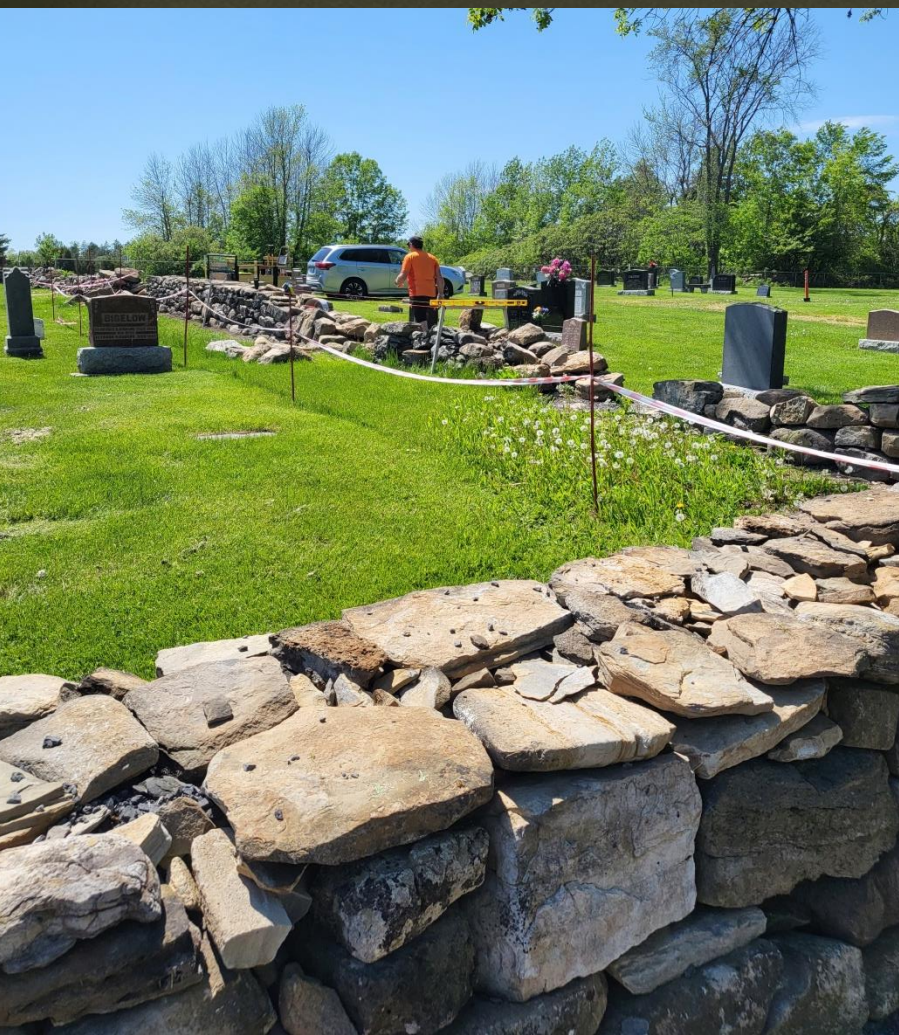
2023 summer work on north wall looking west by Mick
